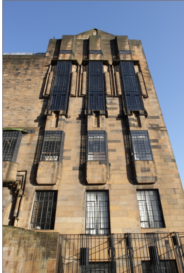
3. West gable facade before fire damage
